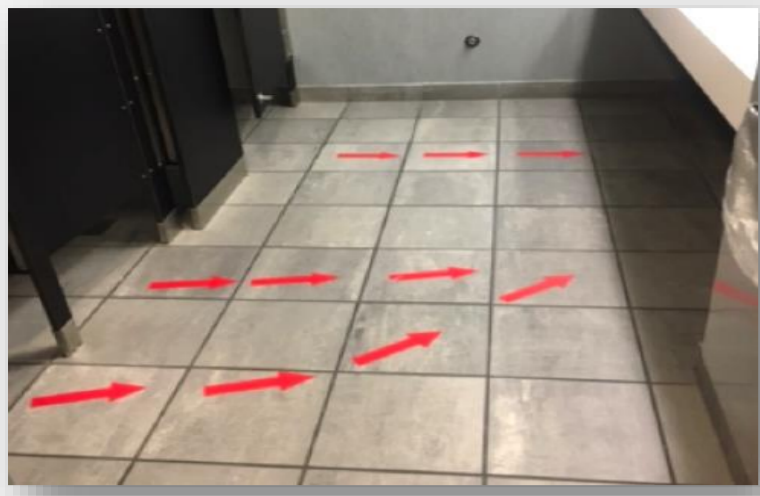
ARROWS ON RESTROOM FLOORS
